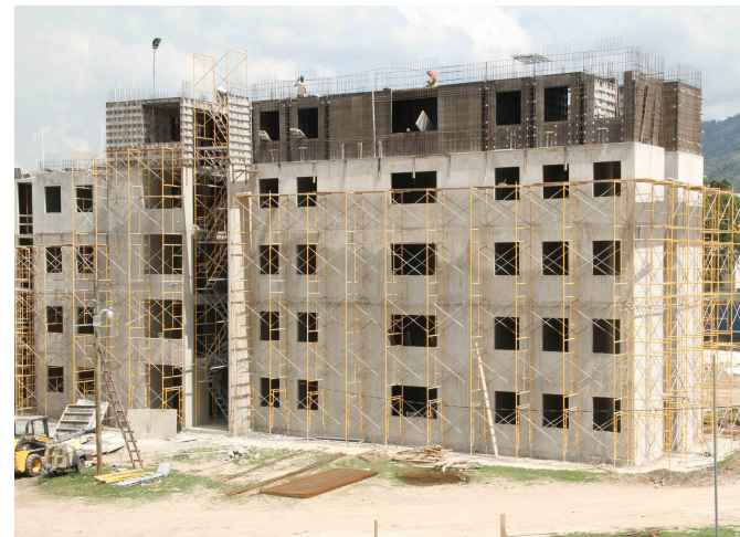
All formwork done without crane.
