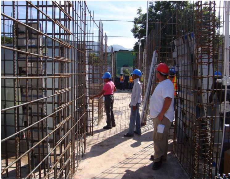
Day 1 - On-site support provided through the first month of construction
