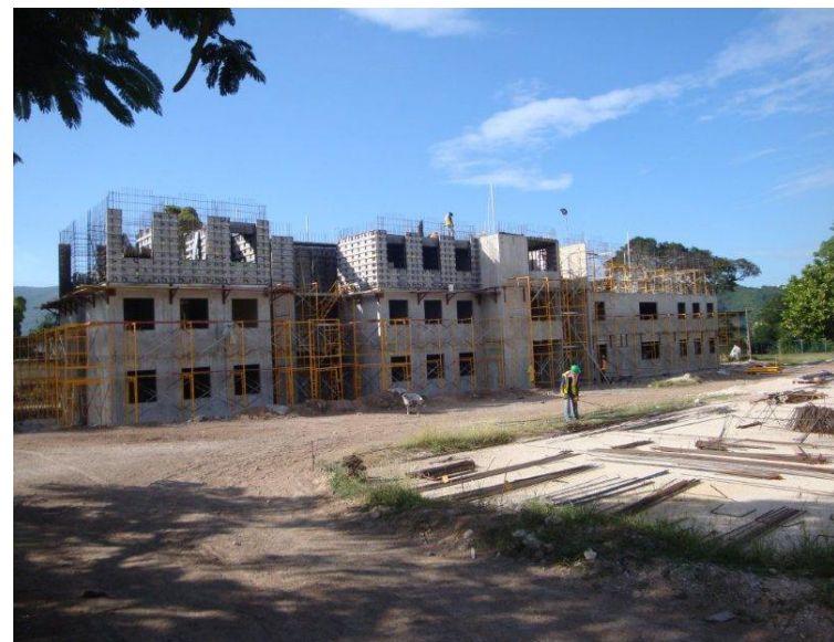
From unpacking of form to first pour was 3 days
