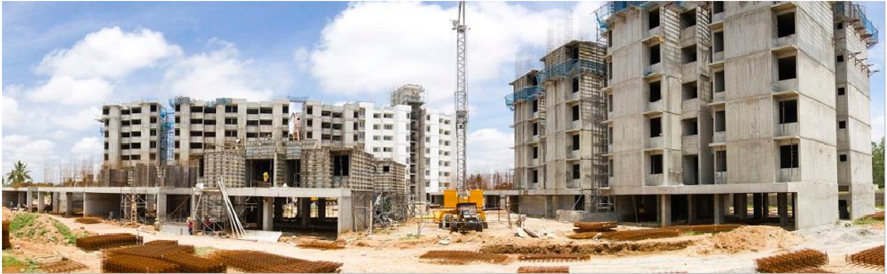
Fast 30 Day Shell Construction
